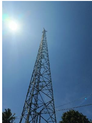
Figure 1. Green Field SST – 3 Legs BTS Tower at Tiirto Yudo Village by PT. Protelindo – Indosat Company
