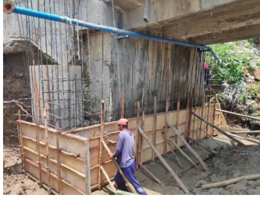
Gambar Pekerjaan abutment
