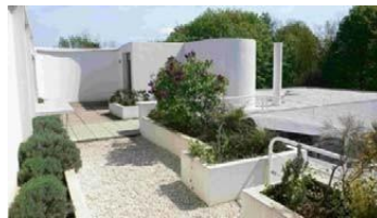
Gambar 14 Roof Garden (Atap Taman)
